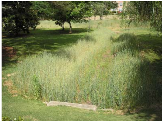
ASHLEY WOODS HOMEOWNERS ASSOC. OUTFALL RETROFIT, VESTAVIA HILLS
