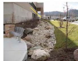
Dry rock Swale
