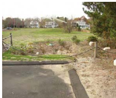
A two cell design with forebay would have worked better for this site.
