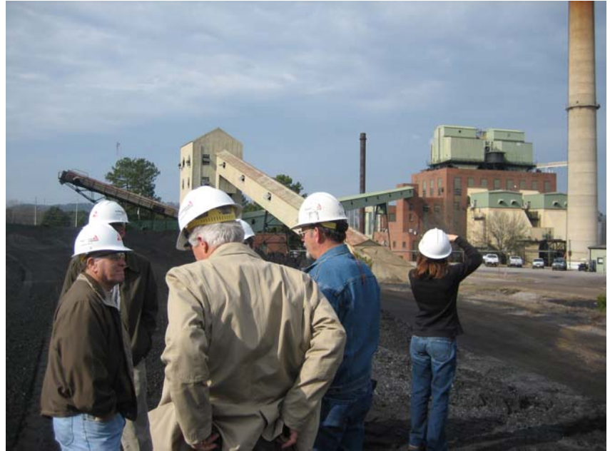
Figure 3 Coal Storage Area - Gadsden Steam Plant
